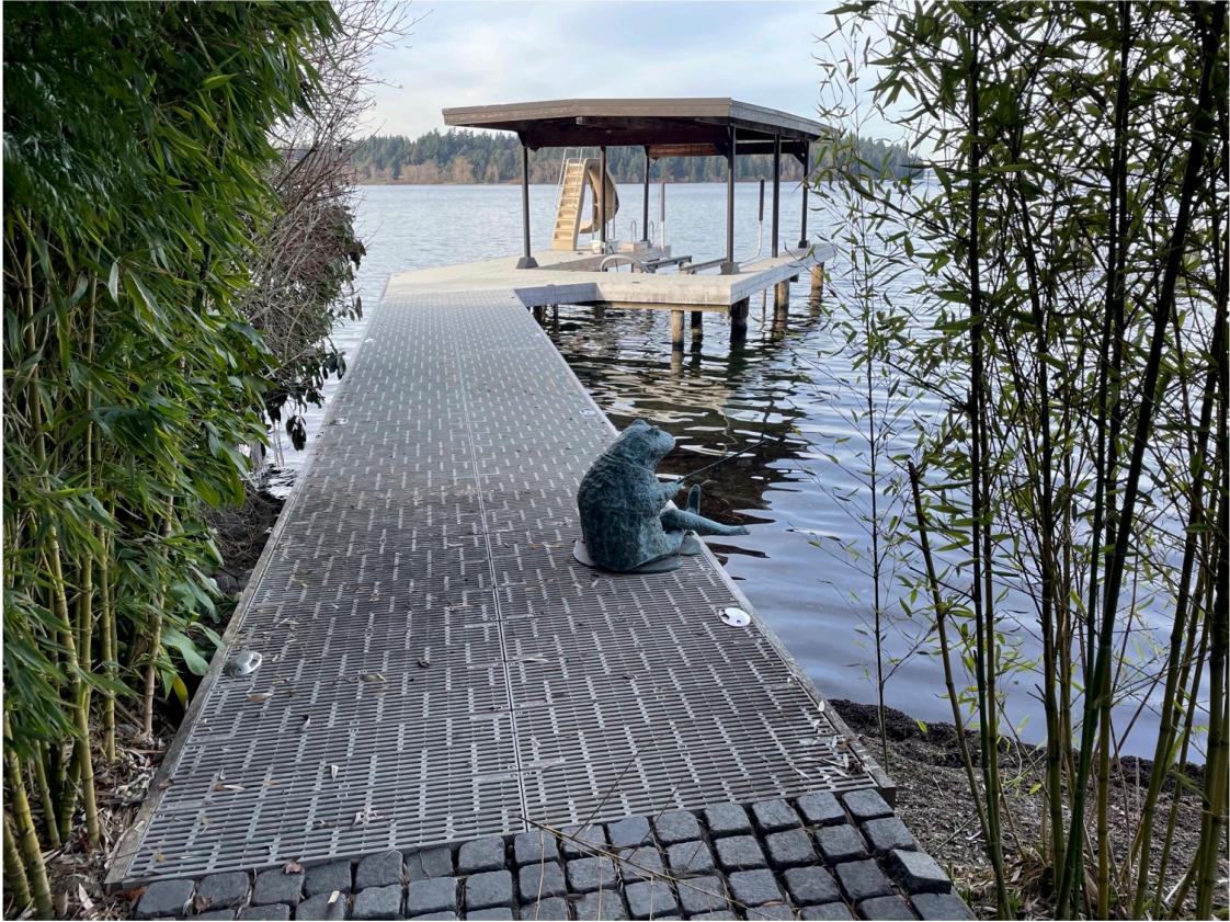
Photo 1 - Existing dock looking waterward.
