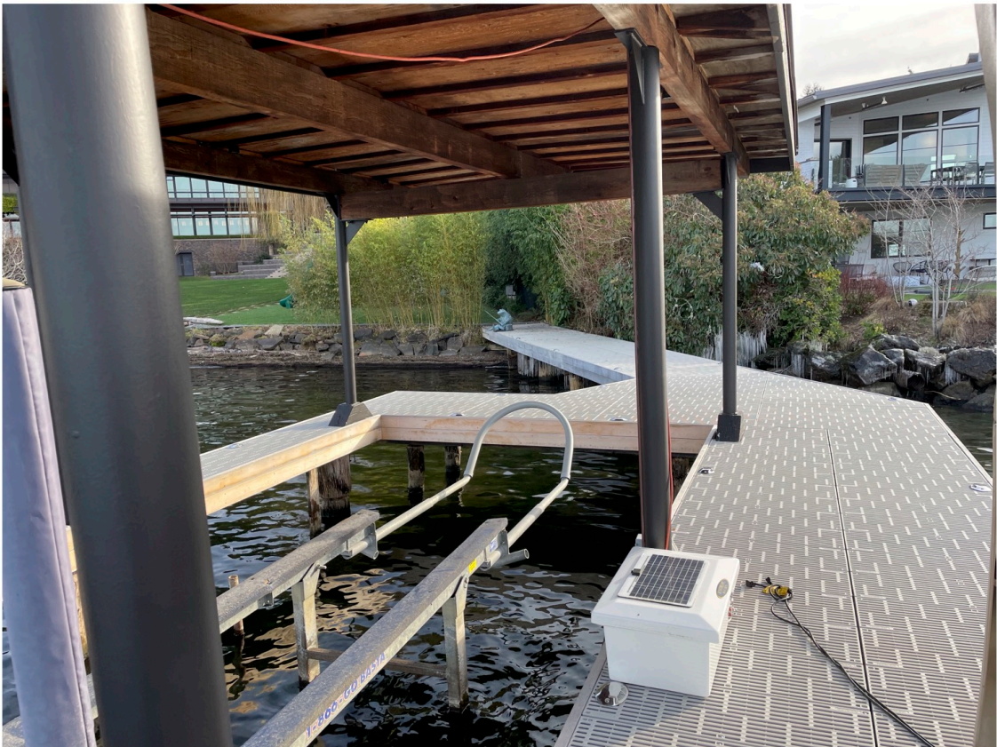
Photo 2 - Existing dock looking landward.
